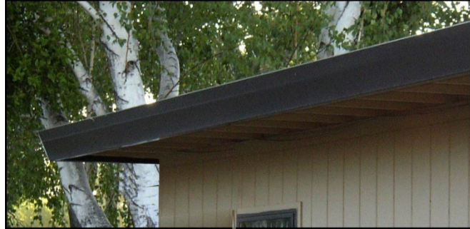
(Roof flashing same color as fascia)
