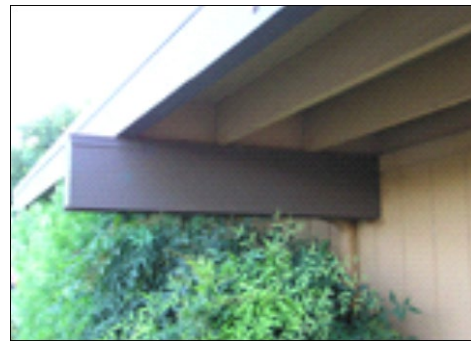
(Beam restoration after dry rot repair)
