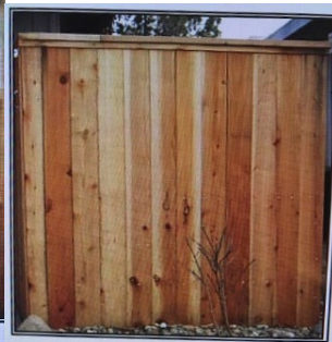
Capped 1"X6" boards)
