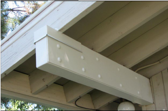
(Beam restoration after dry rot repair)
