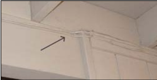
(Cables tied together & run along base or under eaves)
