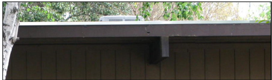
(Roof flashing should be same color as fascia)
