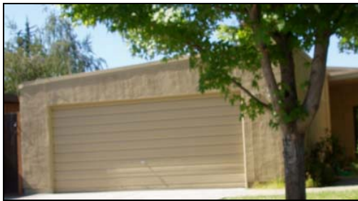
STYLE 1. Half-plex with raked stucco body; roofline with narrow fascia, no overhang and no exposed beams; sliding patio door (out of sight on right); (garage door is not original)
