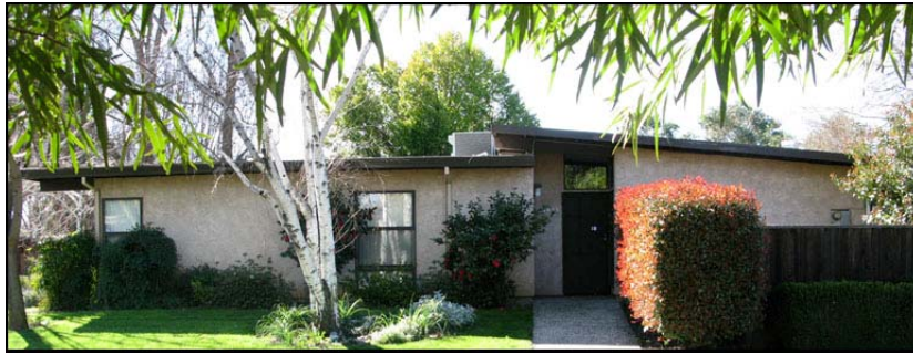
STYLE 9. Half-plex on corner lot with stucco siding; wide fascia, overhang and exposed beams; tall vertical windows; both sloped and flat rooflines.
