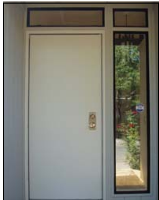
Front door transom and side windows
