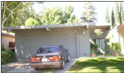
STYLE 2. Single family house with vertical wood siding body; wide fascia, overhang, and exposed beams; 2-car garage; sliding patio door
