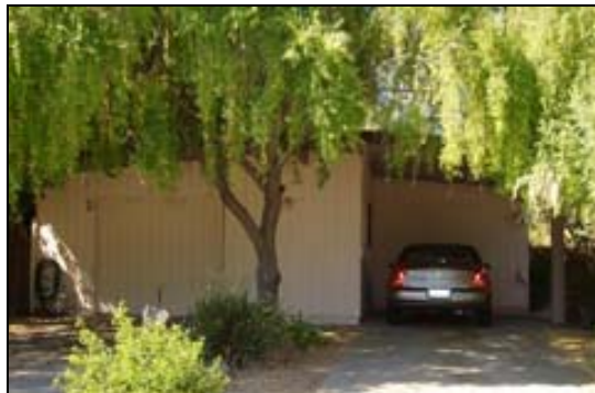
STYLE 7. Single-family house with vertical wood siding; wide fascia, overhang and exposed beams; unique in that it has both carport and garage and no front windows
