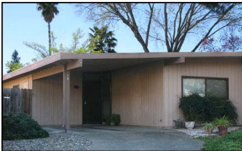
STYLE 5. Half-plex with vertical wood siding; wide fascia, overhang and exposed beams; horizontal bedroom window; carport; slightly sloped roofline
