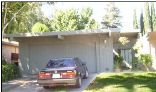
STYLE 2. Single family house with vertical wood siding body; wide fascia, overhang, and exposed beams; 2-car garage; sliding patio door
