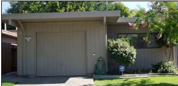
STYLE 4. Half-plex with vertical wood siding; wide fascia, overhang, and exposed beams; front door along left side; horizontal bedroom window; original garage door
