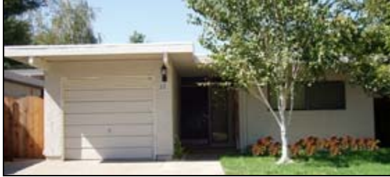
STYLE 3. Single-family house with stucco siding; wide fascia, overhang, and exposed beams; horizontal bedroom window; (garage door is not original)
